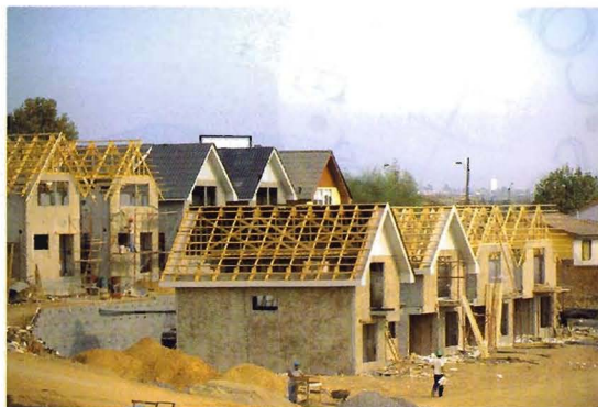
Figure 2 right: 'Jardines del Sol 3' in Val Parasio, Chile – tilt-up wall construction using Barchip Macro synthetic fibre.
